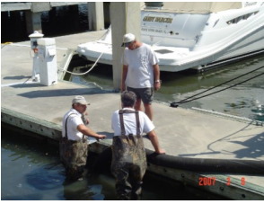
City Crew removing silt under Plaza Dock in 2007
